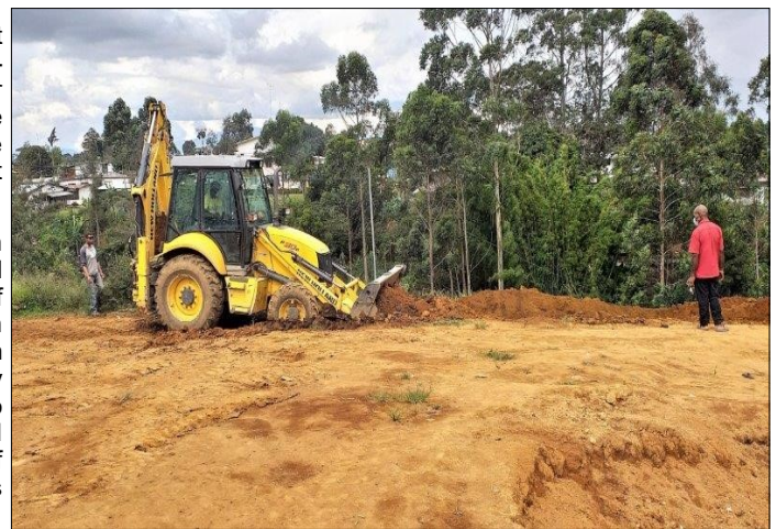
A backhoe clearing the area for a new incinerator shed to be built.
