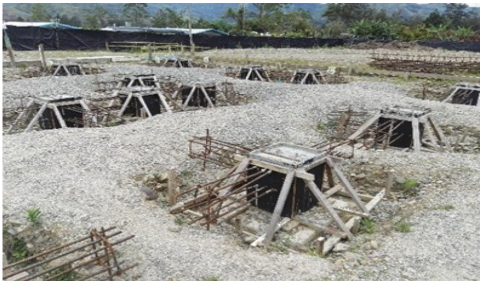
Pictured above are structural footings constructed during the early stages of the construction phase at the new Kotna District Hospital.
