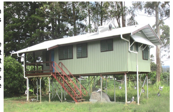
Pictured above - A staff house at one of the CHPs nearing completion and left, a clinical building also nearing completion.
