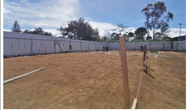
Pictured top - earthworks being carried out while above right, profiling commences and left, one of the many containers with building materials on site.
