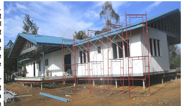
The new urban clinic at Wagbel nearing completion
